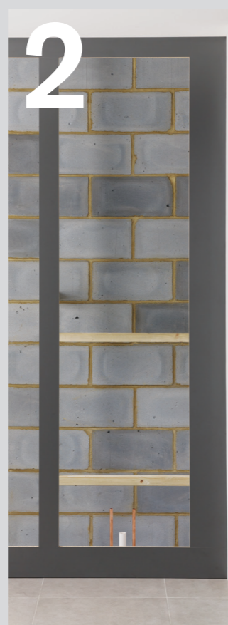
02 Fit base flashgaps to the site frame followed by vertical, horizontal and top flashgaps.
