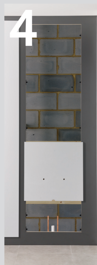
04 Drill or cut out for sanitaryware.
