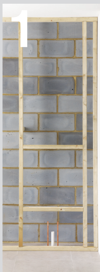
01 Install timber-frame (supplied by others).
